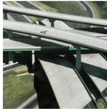
1987: Since 1980, bidding alternate designs has gained in popularity and has allowed steel to be more competitive, resulting in such structures as the I-20/I-459 Interchange in Jefferson County, Ala.
