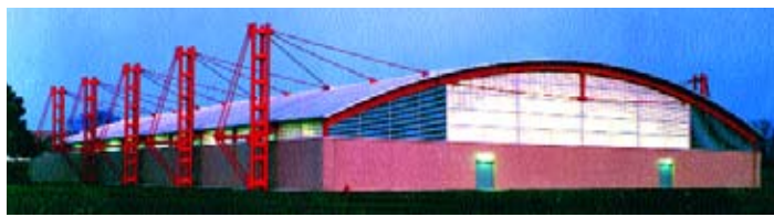
1997: The Nilus West Field House in Skokie, Ill., minimized its internal volume (and therefore the space that needed to be heated and cooled) by moving the structural system outside the building.
