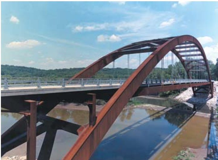
▲ 2001 Prize Bridge Award—Long Span: The Paper Mill Road Bridge in Baltimore County, Md., features a steel box arch.
