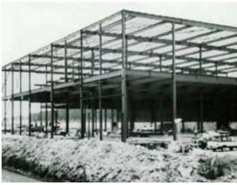
1985: Fast track construction is all the rage; the 172,000-sq-ft Federal Express storage facility in Memphis goes from ground breaking to occupancy in just nine months.
