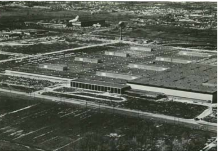
1967: Setting what might be a record for a building of its size, a 2.6-million-sq.-ft Chrysler plant was designed and constructed in just 11 months.
