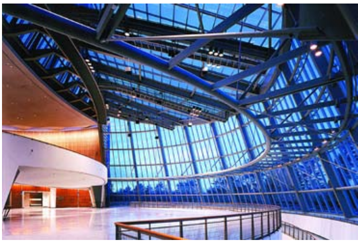
2000: Fire engineering saved $750,000 by reducing the need for passive fire protection of the exposed steel at the Mashantucket Pequot Museum in Ledyard, Conn.
