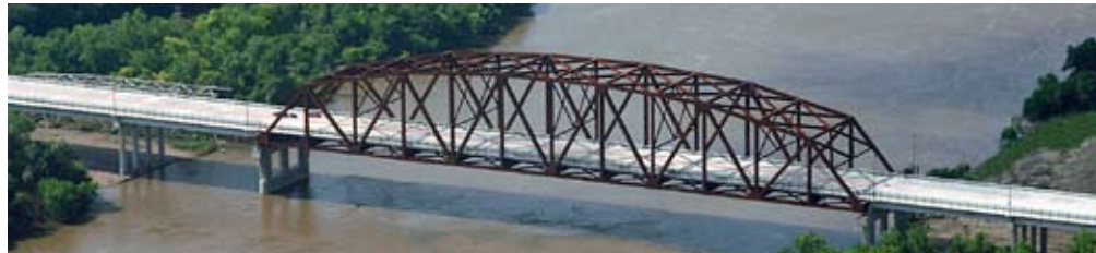
▲ U.S. 275 crosses the Missouri River on the Veterans Memorial Bridge's 624-ft. center span, which provides the Coast Guard-required 600 ft minimum horizontal clearance for navigation.
