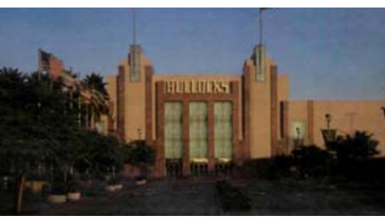
1994: Moment connections provided both long spans and structural stability on the Bullocks department store building in Burbank, Calif.
