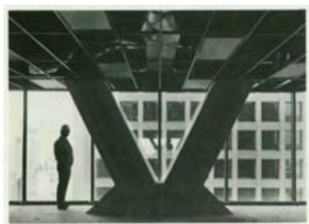
1976: The 56-story First International office building in Dallas features a trussed tube design with diagonal X-bracing and stub girders.
