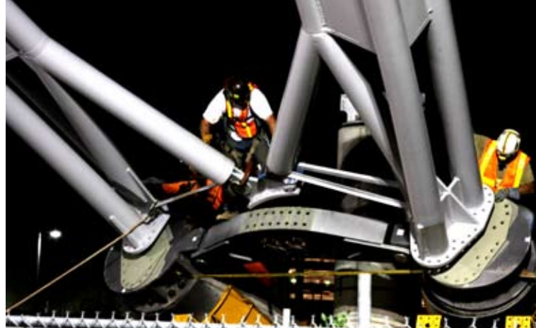
▲ Arches being lowered onto the inclined concrete column supports, prior to being bolted down.
