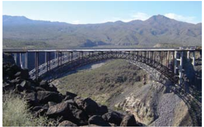
▲ 2007 Prize Bridge Award—Major Span: The Burro Creek Bridge on U.S. 93 between Phoenix and Las Vegas.
