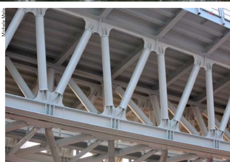
▲ Detail of the reticular spatial structure that successfully combines a lean look with solid seismic resistance.
