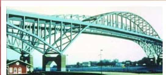
1997: The Blue Water Bridge between Port Huron, Mich., and Sarnia, Ontario, is an early example of the use of LRFD in bridges (it was also designed with all SI units).
