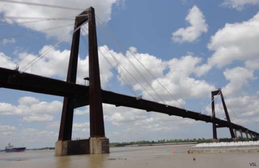
◀ The Luling Bridge, also known as the Hale Boggs Memorial Bridge, is getting new cable stays with a mix of both HDR and friction dampers.
