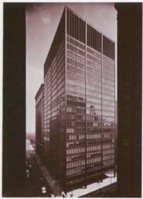
1965: Steel's advantage in office building design is evident in the Continental Center project, which featured 42-ft square bay spacing—a previously unheard of figure in Chicago.
