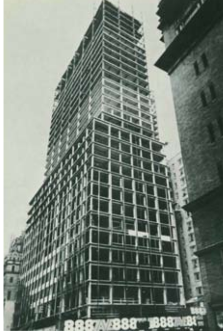
1969: 888 7th Ave. in New York is an early use of composite construction.
