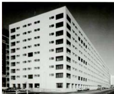
1983: The Barnes Building Rehabilitation team touts their extensive use of computer analysis using STAAD-III.
