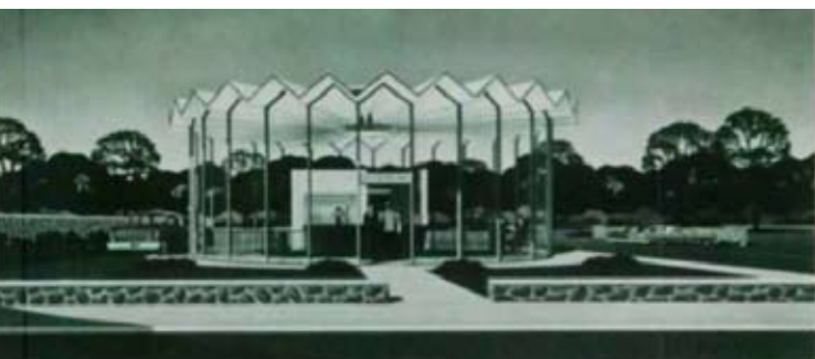
1962: Steel designers are introduced to a new shape when steel tubes make their first appearance in MSC in an article entitled "New Member Joins Structural Family."
