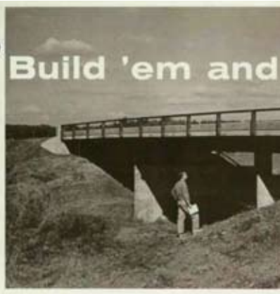
1970: MSC touts the use of weathering steel for short-span steel bridges.
