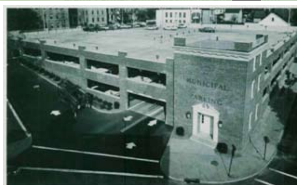
1963: Parking structures were a growing market and AISC showcased several projects using high-strength steel to minimize columns and reduce costs.
