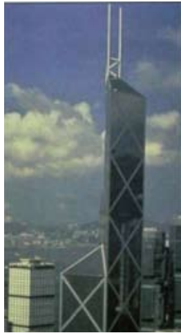
1994: Larry Griffis' T.R. Higgins lecture offered everything you need to know about composite frame construction, using the Bank of China in Hong Kong as one example.
