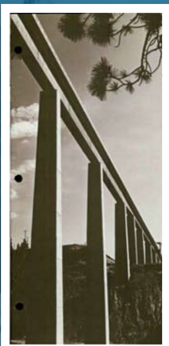
1973: The Latah Creek Canyon Bridge in Spokane is an early example of a steel box girder bridge.
