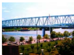
1997: Combining Grades 70W, 50 and 36 on the Central Bridge between Newport, Ky., and Cincinnati allowed the designers to maintain a constant girder depth.
