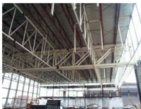
2006: The roof of the old center was salvaged and reused when the Richmond (Va.) Convention Center was expanded.
