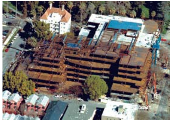
2003: Steel framing dominates the early ranks of LEED-certified buildings, including one of the first Gold projects, the Department of Education Building in Sacramento.
