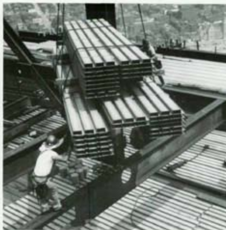
How to Fasten Steel Deck
