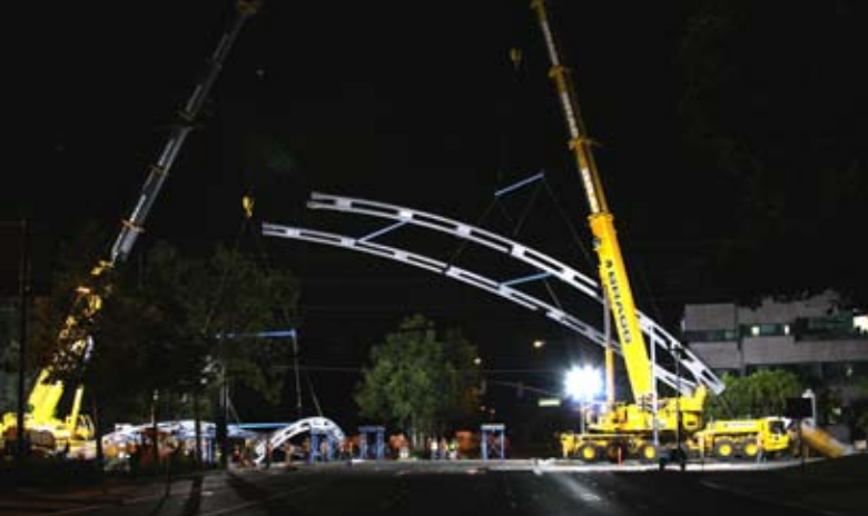
▲ Two arch sections are lifted to their final positions with temporary bracing. They were erected on the first of three weekend night closures.
