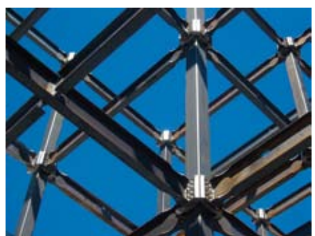
2005: Building 1 at Santa Row in San Jose, Calif., was one of the first to use the proprietary ConXtech system.
