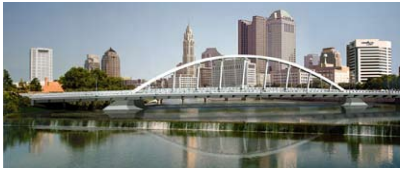
2007: The Main Street Bridge in Columbus, Ohio, is the first inclined single-rib arch bridge in the U.S.
