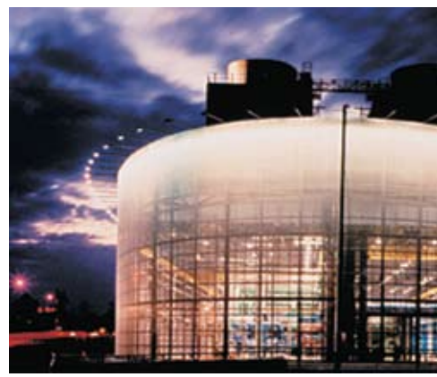
2001: Utilitarian doesn't have to mean pedestrian, as this chiller plant in Philadelphia proves.
