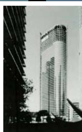
1983: Four Allen Center in Houston is designed as a cirque-ovular building to reduce wind loads.
