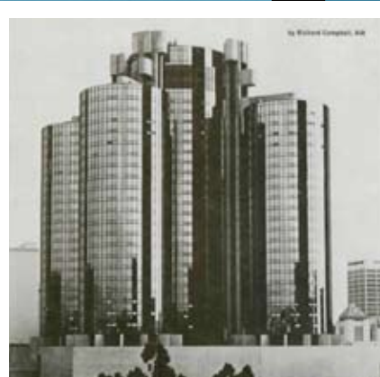
1977: The landmark Los Angeles Bonaventure Hotel features a cluster of five towers, all tied together to meet seismic design requirements.
