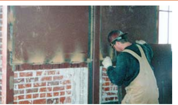
2000: The steel-plate shear wall installed during the rehabilitation of the Oregon State Library in Salem was a precursor to a system that gained popularity later in the decade.
