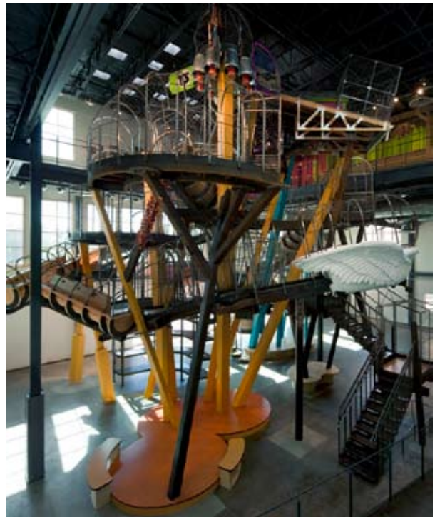
2010: The climbing structure at the Children's Museum in Phoenix required more than 400 bolted connections.
