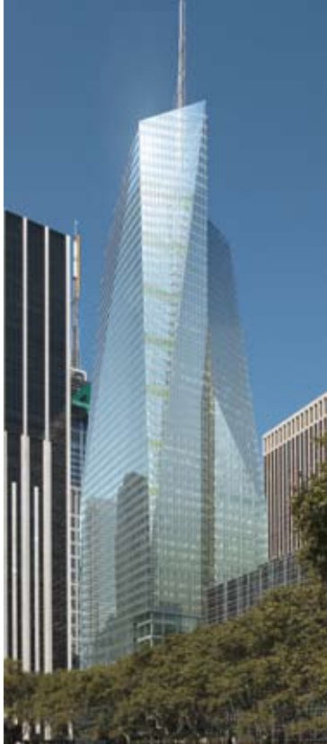
2008: The Bank of America Tower in New York City features 15-ft cantilevers to create column-free executive offices.
